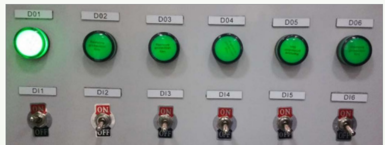
Fig.3: External emergency switches
